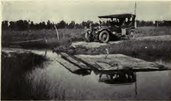
This situation, encountered in Montana, necessitated the taking apart and reconstructing the bridge. Laborious and slow but counted as all in the day's work
